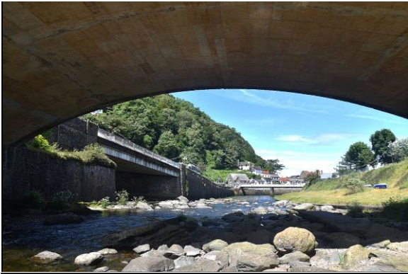
River and bridge at Lynmouth. John Batt
